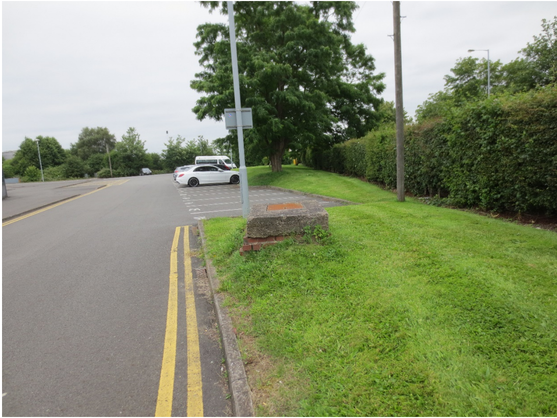
Photo 1: Pirrelli Stadium - Existing manhole SK25243901
