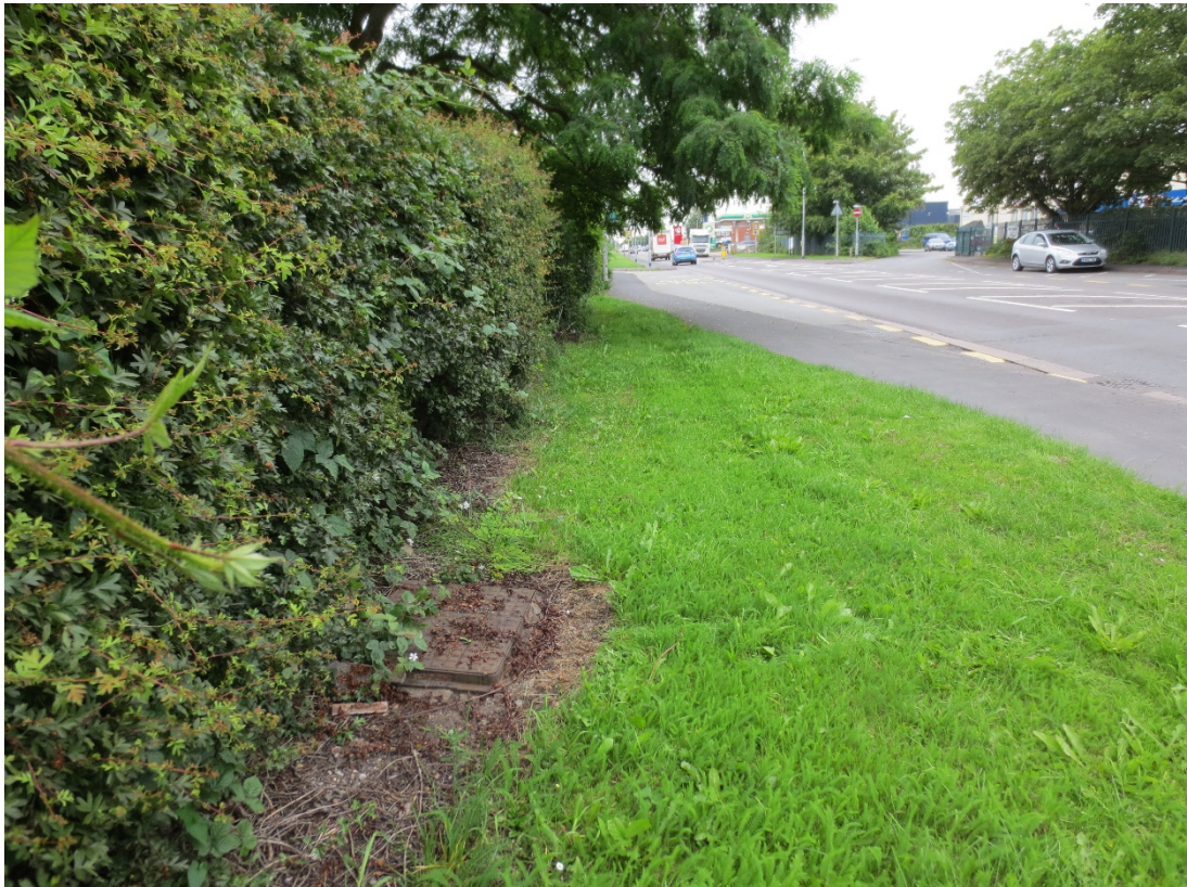
Photo 2: Derby Road – Proposed requisition manhole location
